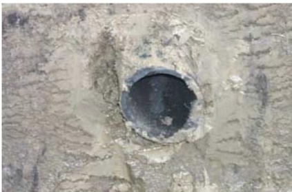
FIGURE 3-7. 100mm (4 in.) Clay Excavation @ 1 day
